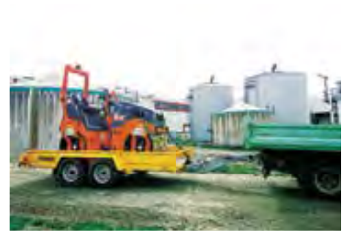
9h00 Arrival at a biogas plant for a compaction work.
